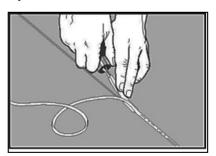
Trim with the chamfering-knife for Granit Multisafe/Optima Multisafe or equivalent. If the raised studs of the embossed pattern are too close to the seam area, cut them off before trimming of the welding rod.
